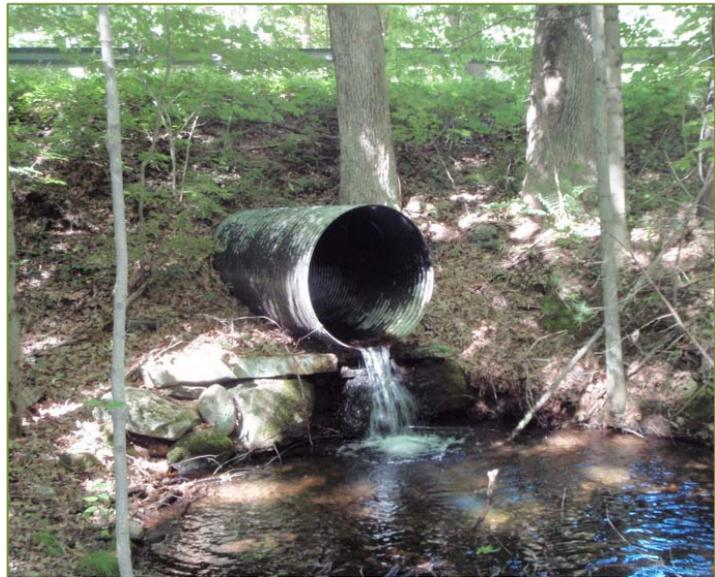
*A “perched” culvert in Union, CT. This is an example of a barrier to potential fish movements in a small stream.*
